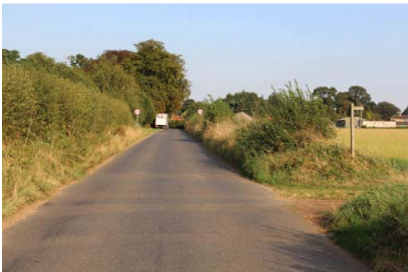
Rectory Lane, North Runcton. Road widening would result in hedge loss.
