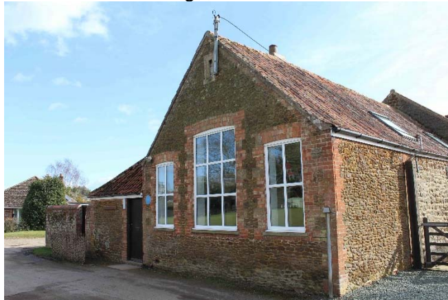
North Runcton Village Meeting Place, School Lane.
